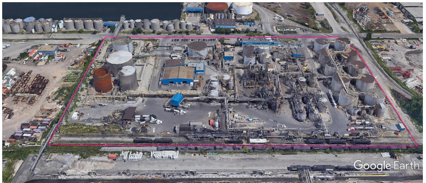
Figure A2: Site-Wide Aerial View 2
