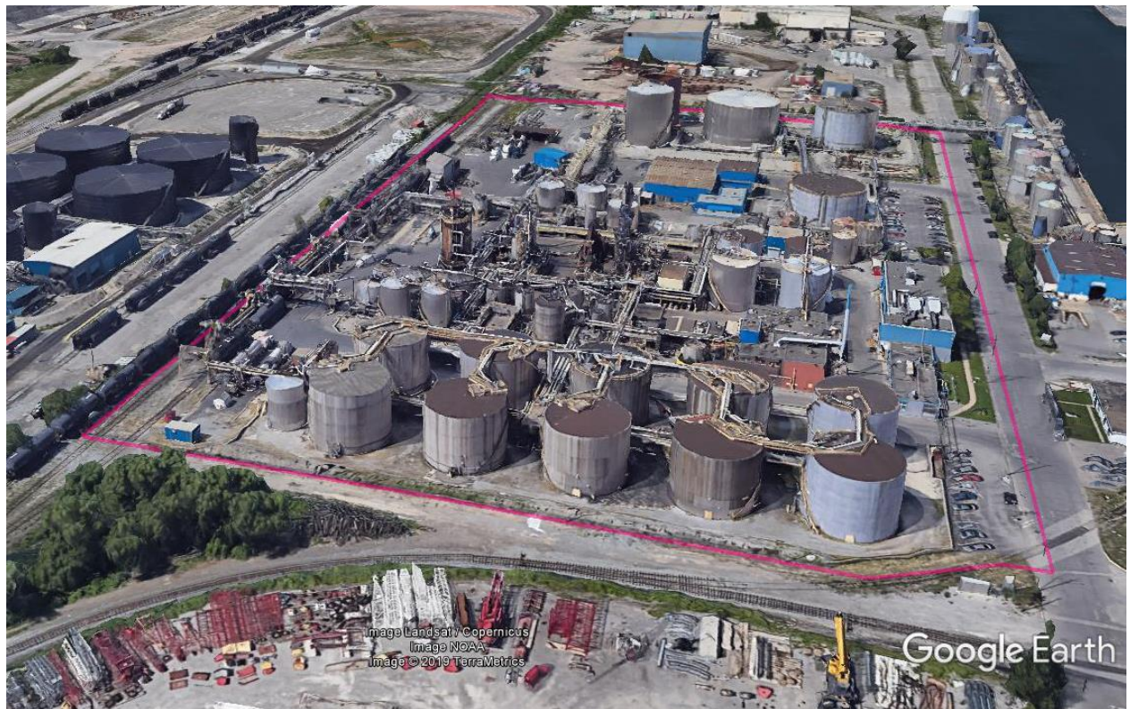
Figure A1: Site-Wide Aerial View 1
